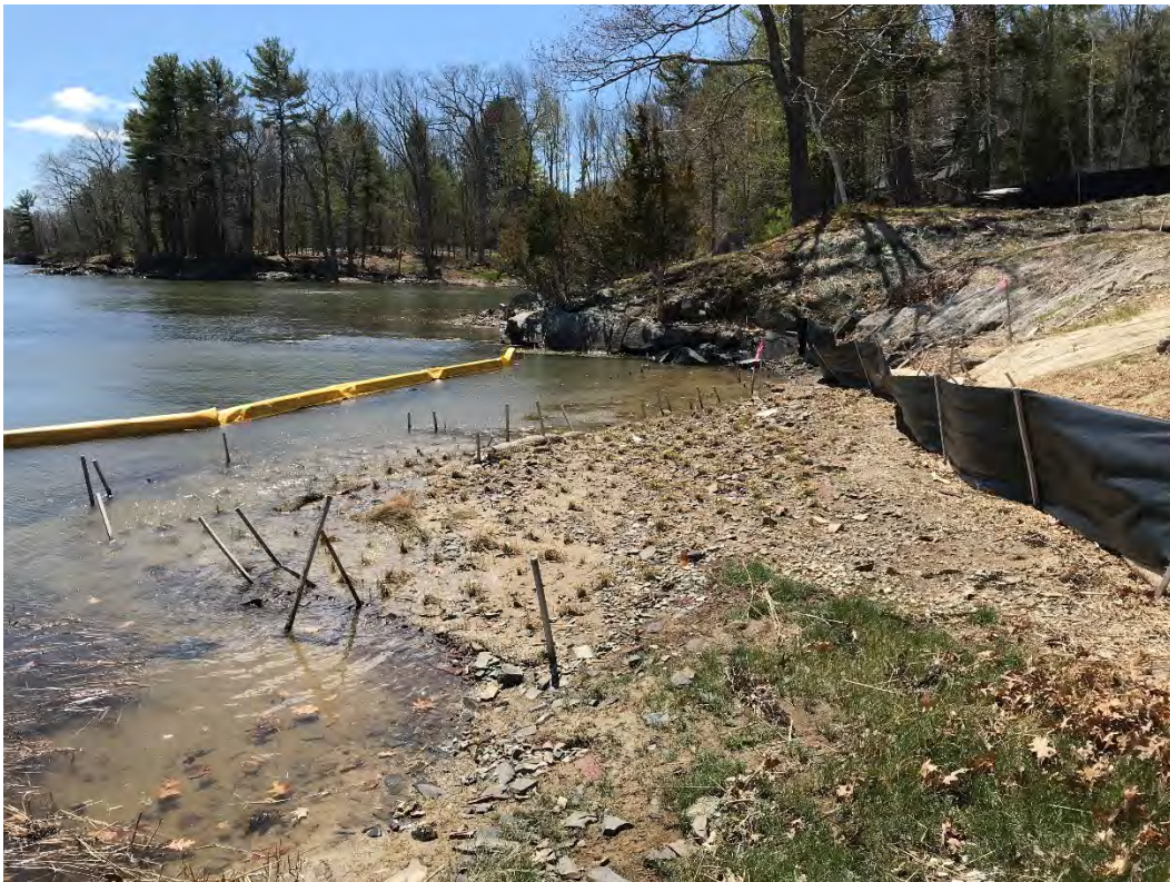
Fig 4: Toe of the slope and salt marsh restoration at the west side of the bay. Viewing south. (04-26-21)
