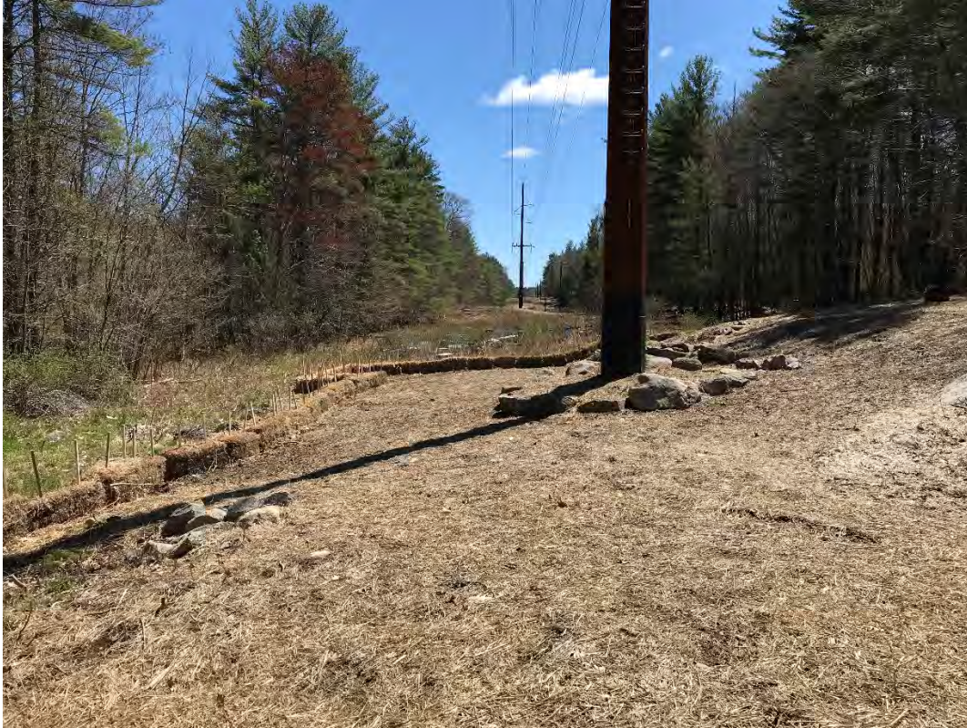
Fig 5: Str. 89 work area. Viewing southeast. (04-26-21)
