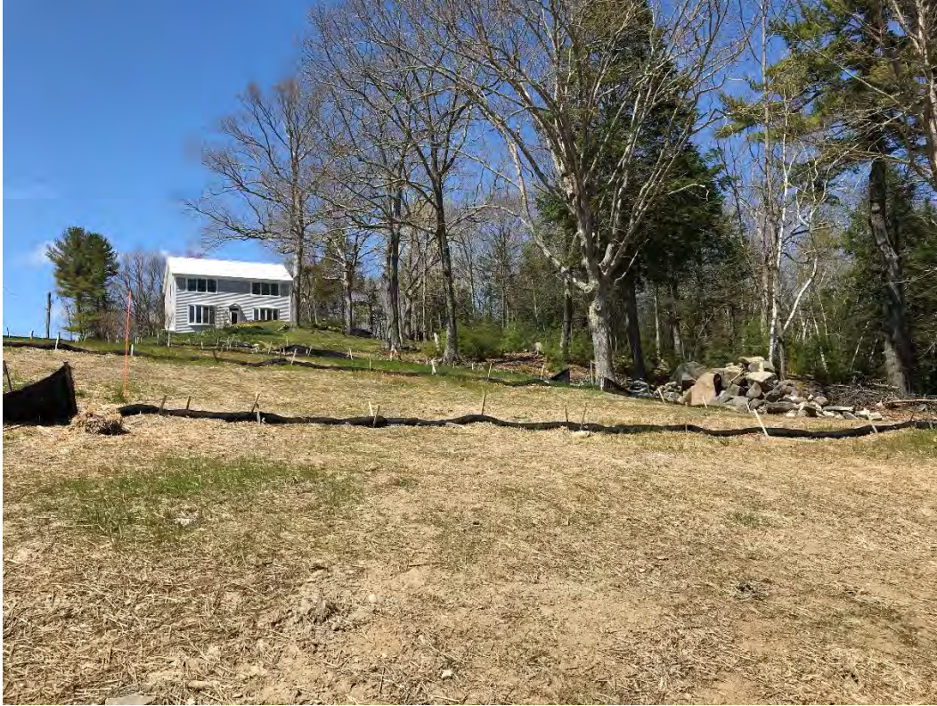
Fig 3: Slope above the cable house at the west side of the bay. Viewing northwest. (04-26-21)
