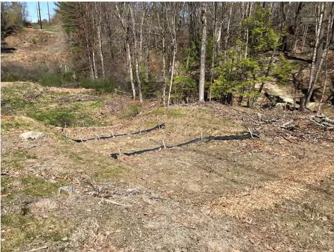
Fig 8: Lower portion of slope between Strs. 28 and 29. Viewing northeast. (04-26-21)
