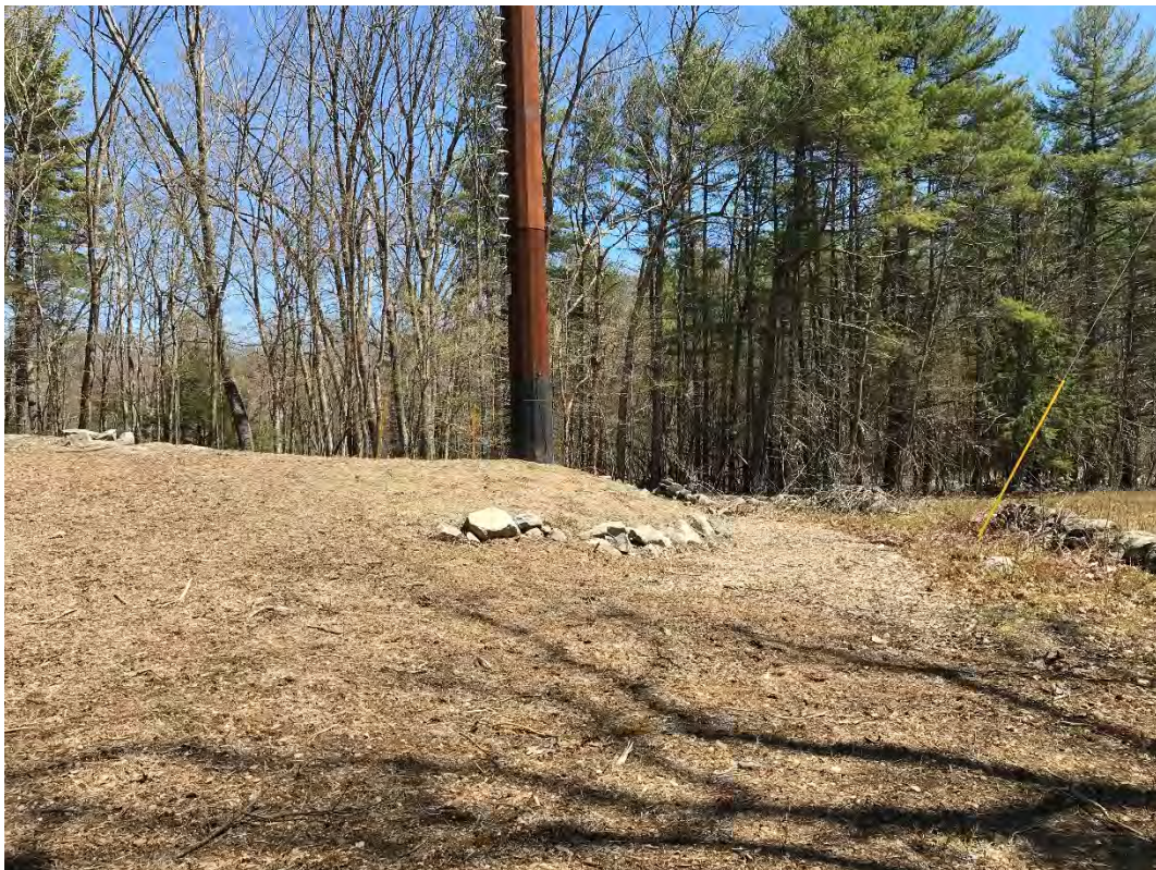
Fig 6: Str. 90 work area. Viewing northeast. (04-26-21)
